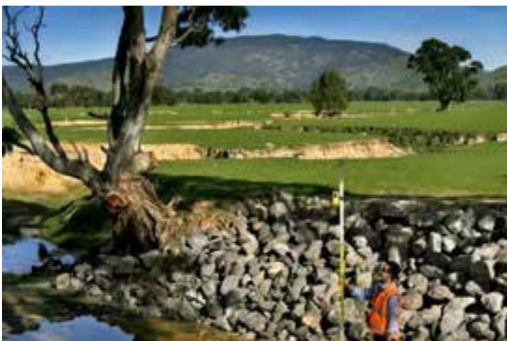
Newly constructed rock chute in a tributary of Nowhere Creek. (Photo: D Fletcher)
